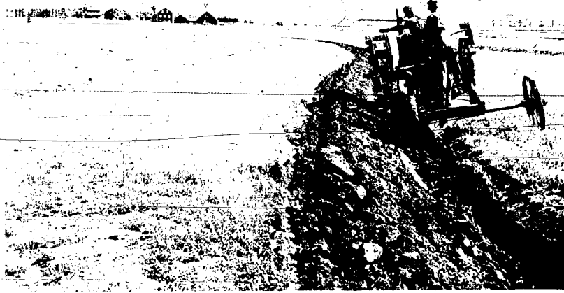
Farmers used to make their own terraces. This Humboldt area landowner in 1936 used his farm tractor with a six-foot blade to build pasture terraces. (Soil Conservation Service Photo)
